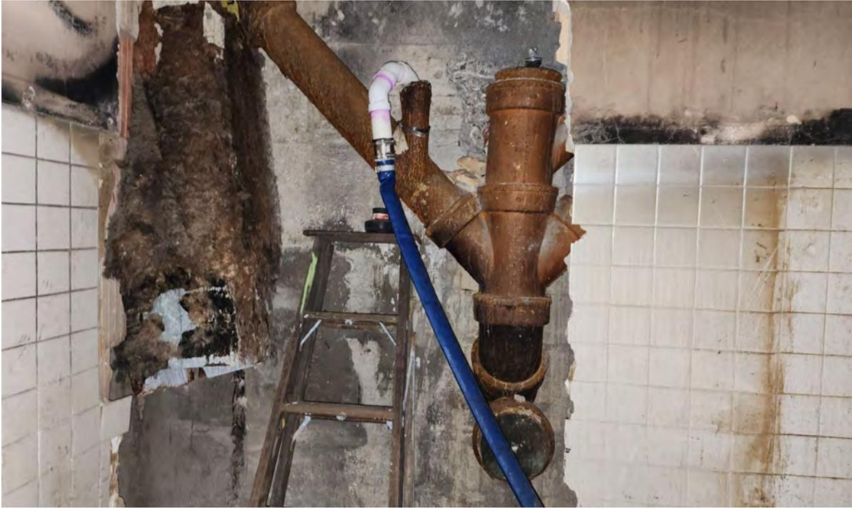
Basement Level: Existing storm service leaving the building. Discharge hose from the temporary sump pump shown discharging into an open pipe fitting.
