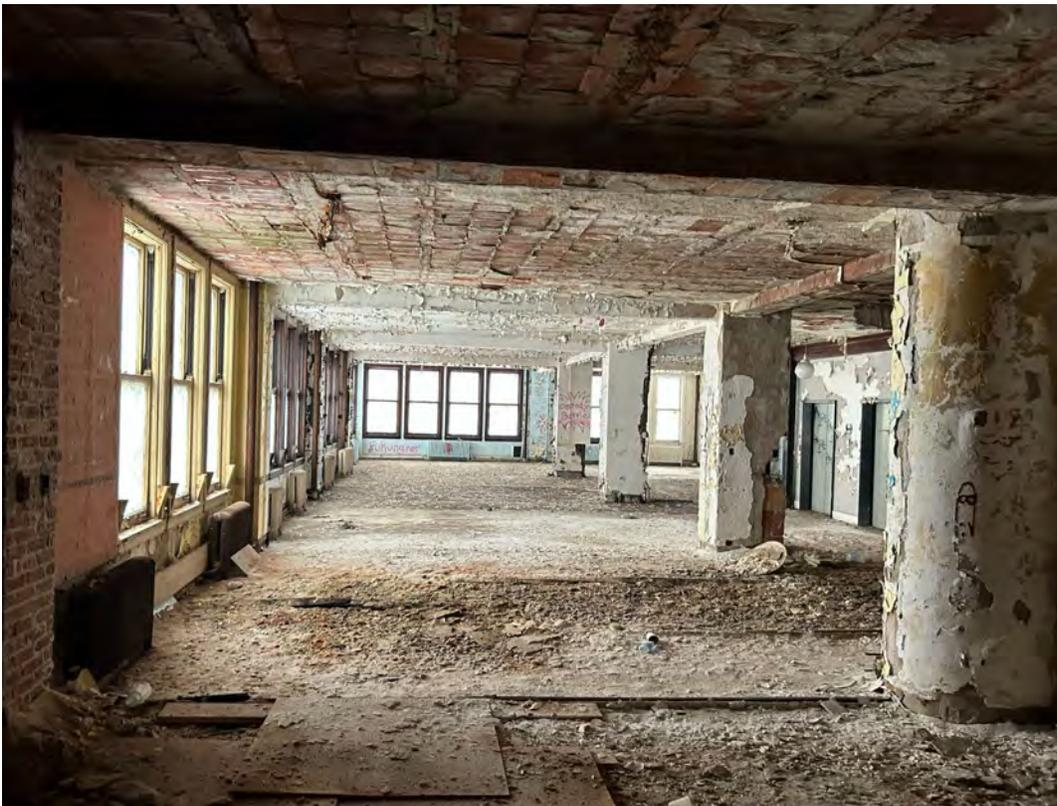
Superstructure: Typical upper floor layout and clay tile arch floor system, looking east
