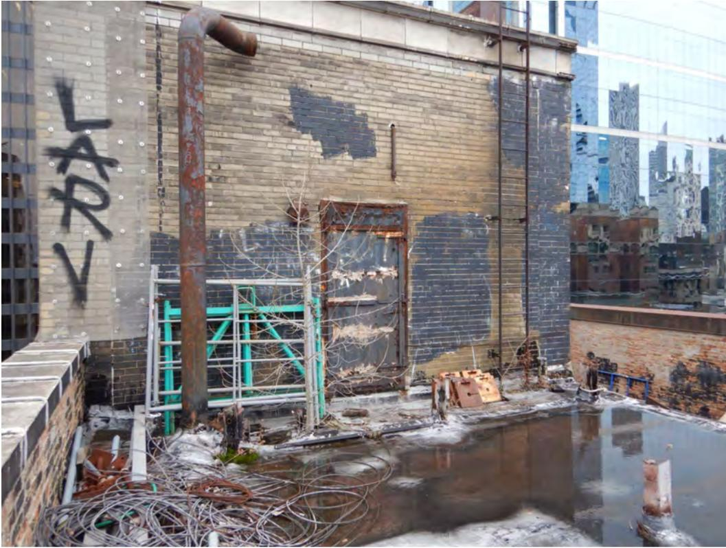
Upper flat roof with ponding water and vegetation growing from roof
