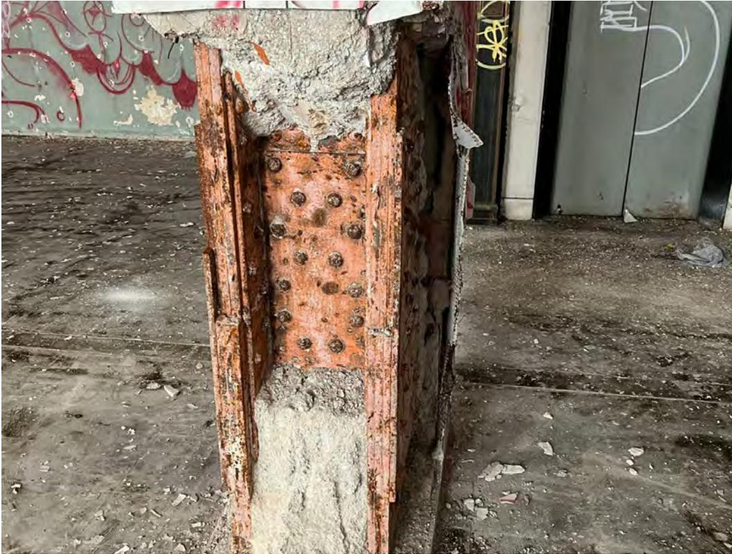
Superstructure: Previously removed concrete encasement on steel column
