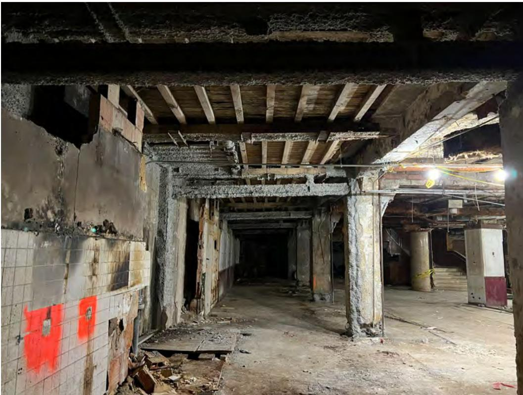
Ground Level slab from below: Vaulted concrete slab at north sidewalk (wood formwork left in place)
