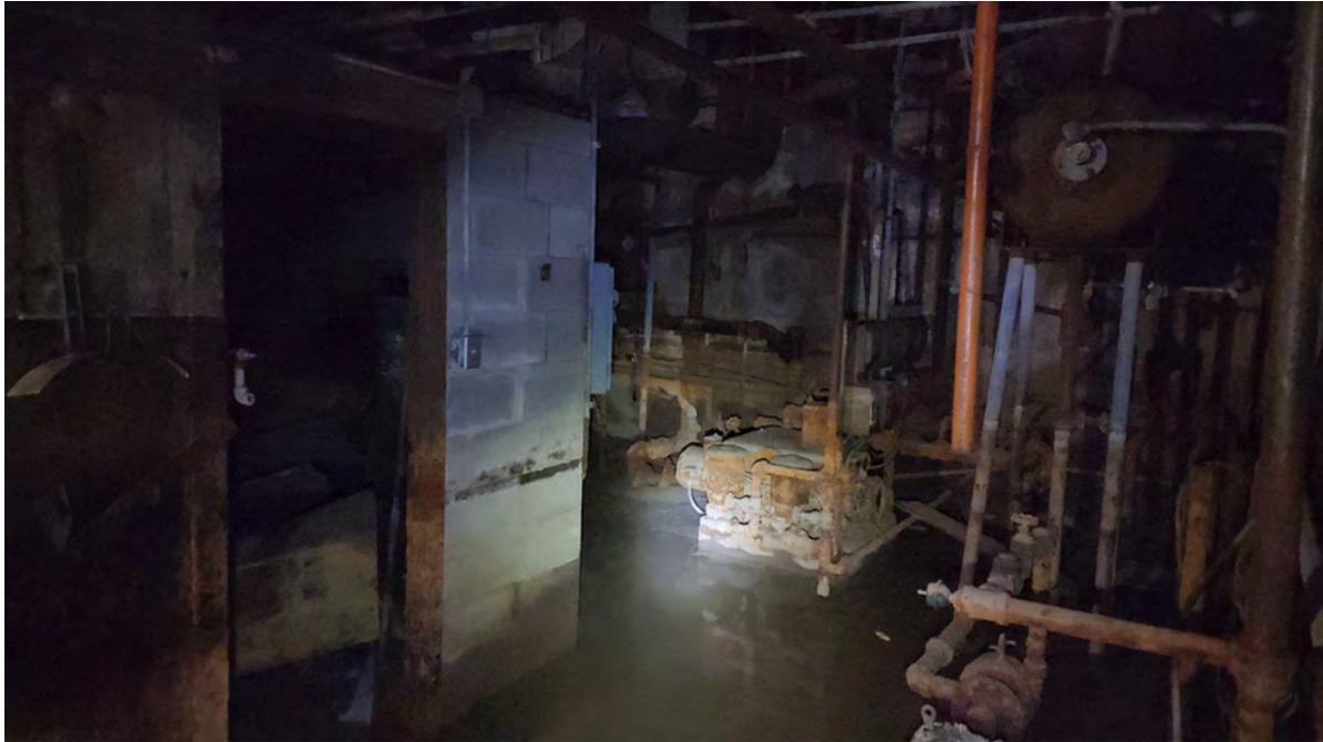
Basement Level: Mechanical and Plumbing equipment in flooded area of the basement. The water ponding is several inches deep.
