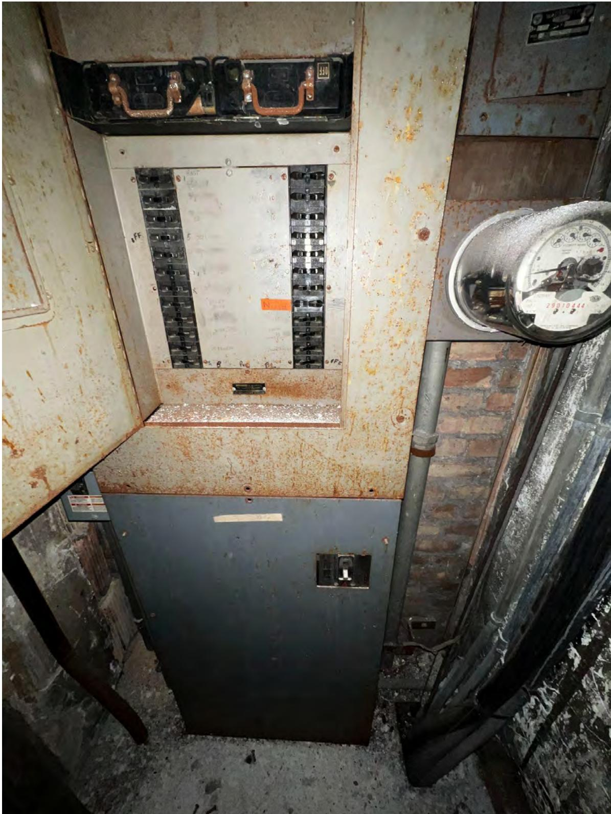
Upper floors bus duct disconnect, panel, and separate tenant metering
