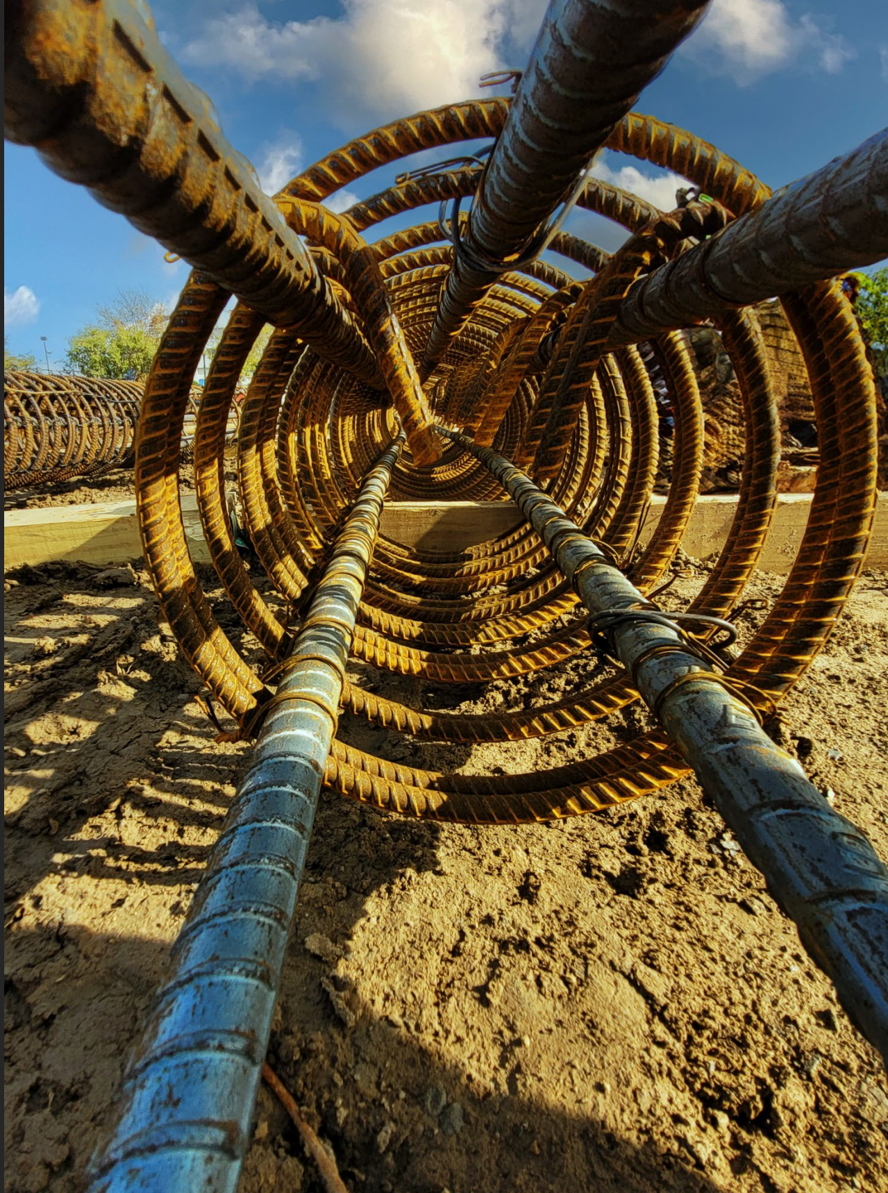
Figure 13: U.S. Courthouse Structure Greenville, MS
